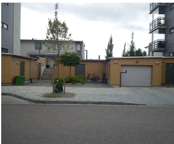
Parkeringsgarage under gårdsmark, Gävle
