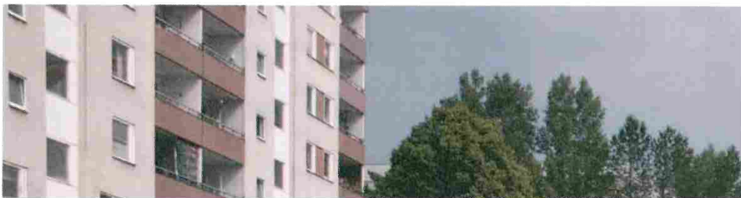
Fornbacka - part of the building stock undergoing renovation
