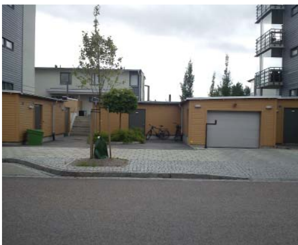
Parkeringsgarage under gårdsmark, Gävle
