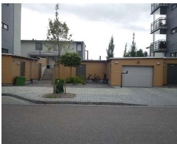
Parkeringsgarage under gårdsmark, Gävle
